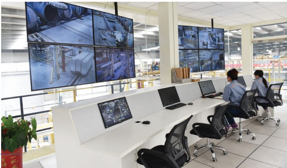
Fig. 8: Central control room.
